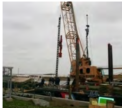
Figure 12-4 Hoisting Hammer and Lead
