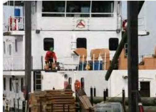
Figure 12-6 Cross Deck Winch Easing Out Pile
