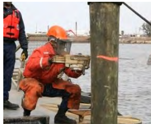
12-8 Cutting Pile Top
