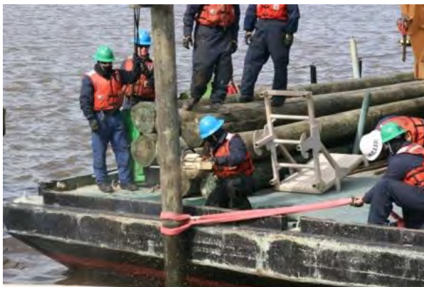
12-7 Cutting Pile Top
