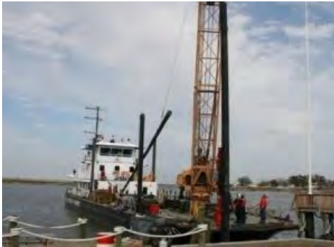
Figure 12-5 Crane Hoisting Pile
